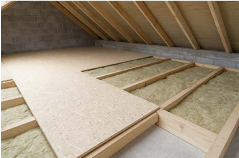
esb panels are the better choice for ceiling panels in the attic due to their more favorable vapor permeability.
