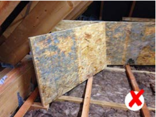
Vapor-tight panel materials are not a good solution for attic floors, as they can lead to mold formation.
